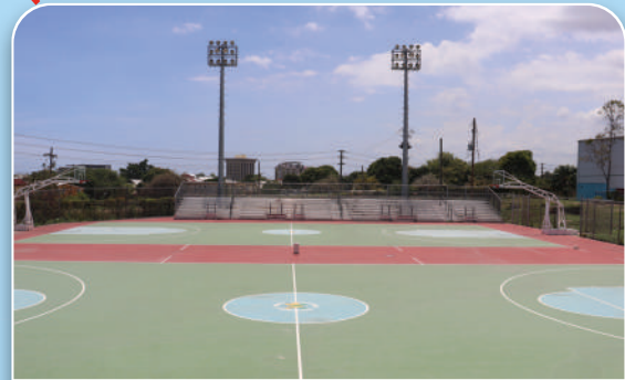
Lighting – National Stadium Basketball Courts, Kingston
